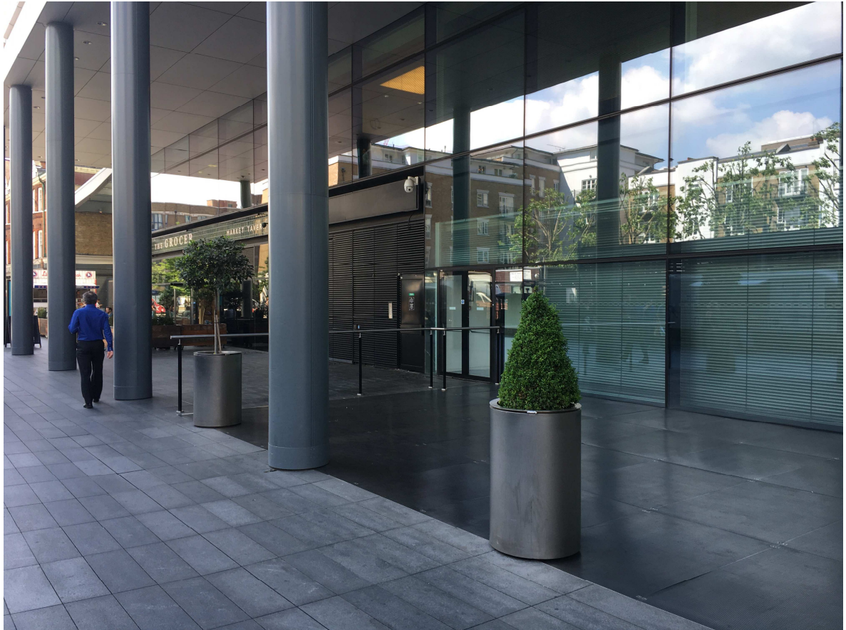
Image 4 – Lamb Street as existing (looking south-east)
